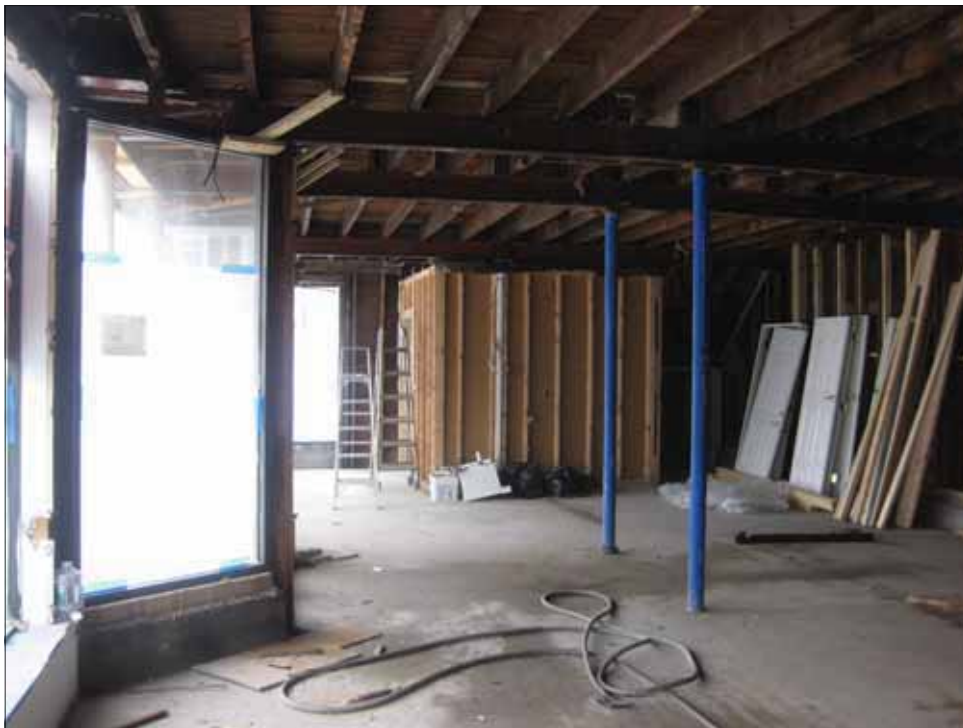
Interior pictures of the ground floor
