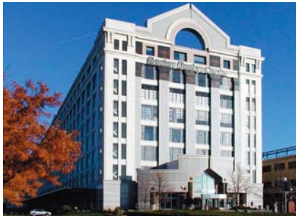
One Design Center, Boston NAI Hunneman leased 30,000 s.f. of space to the Boston Beer Company at the Boston Design Center, which was recently purchased by Vornado
