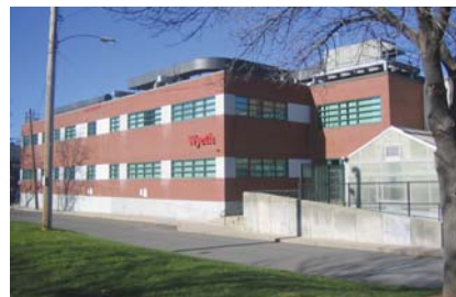
85 Bolton Street, Cambridge New to the tightening Cambridge market is this 43,000 s.f. Class A office and lab building at 85 Bolton Street. Available for sale or lease
