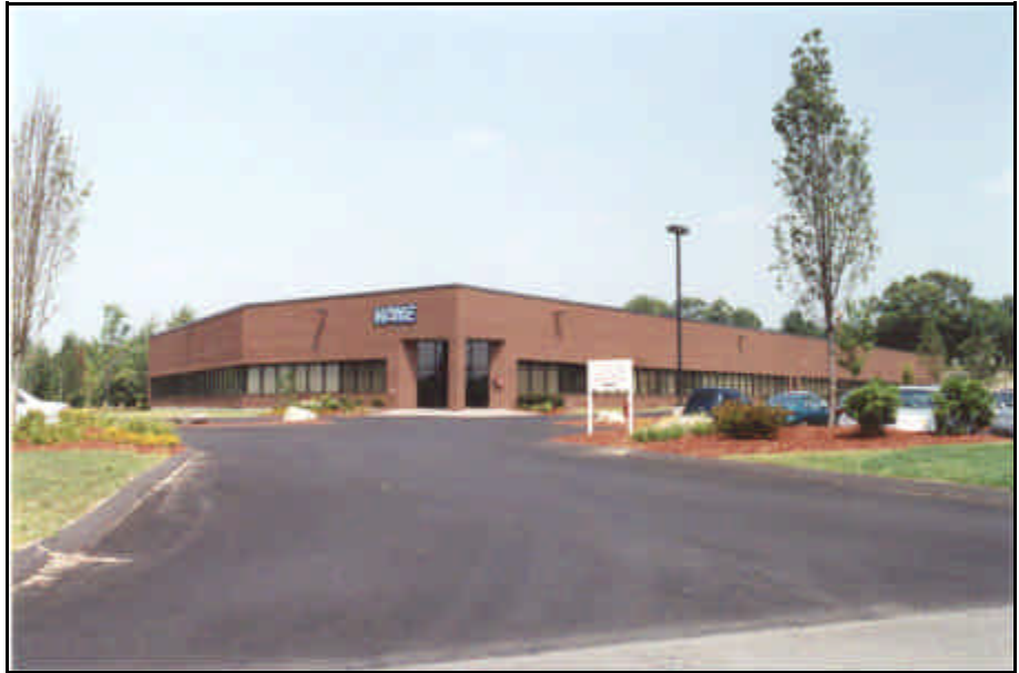
Recently completed Building 7 at 101 Billerica Ave. in North Billerica is leased to Kaye Instruments, a subsidiary of Spirent PLC. This business park has expanded considerably in recent years, confirming demand for R&D (flex) space in an attractively landscaped setting.
