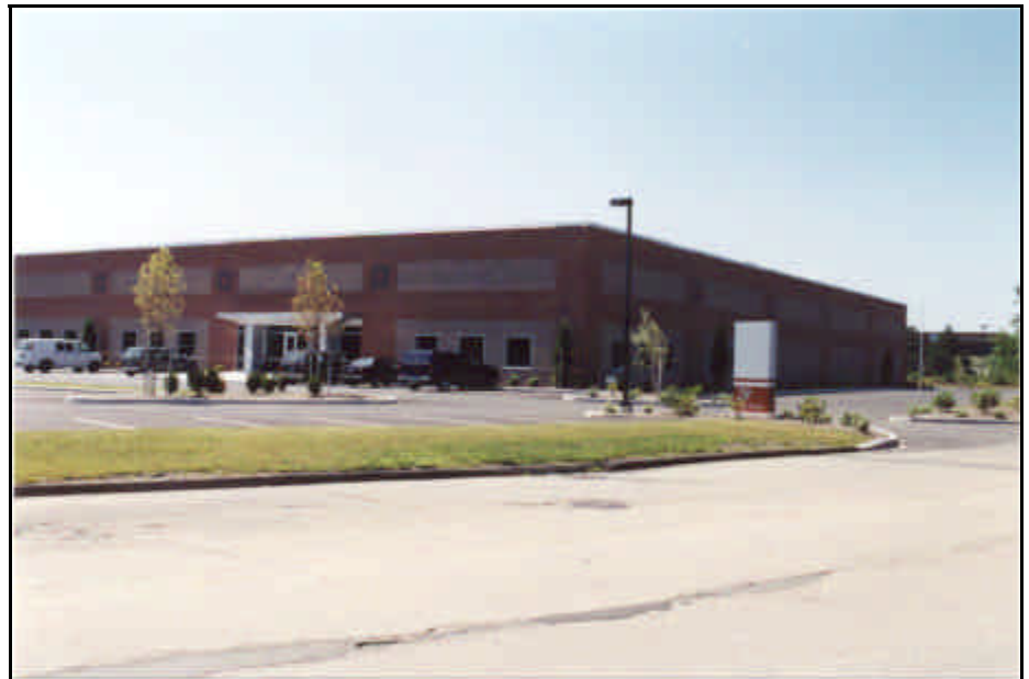
Completed early this year, 20 Dan Road, Canton, is a 104,000 SF flex building constructed by Conroy Development. A similarly-sized flex building nextdoor at 10 Dan Road was completed last fall.
