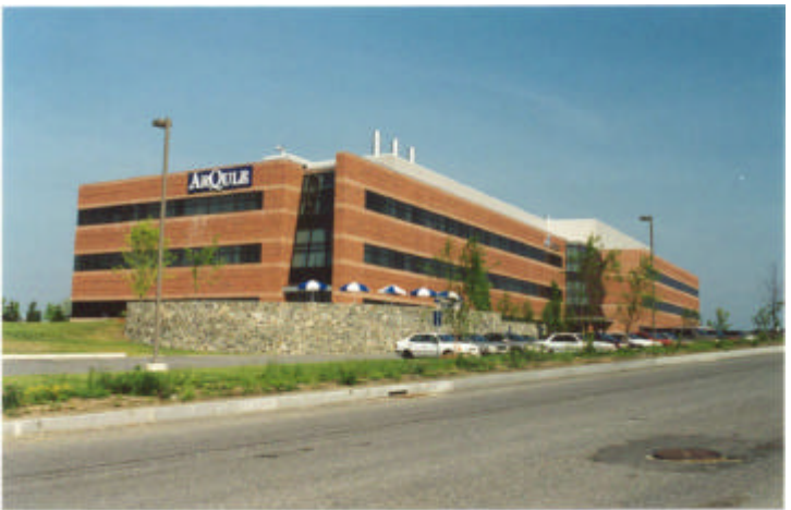
ArQule, Inc. exercised a purchase option on its new office/lab facility in Woburn near the end of last year, as well as on 5 adjacent acres of land.
